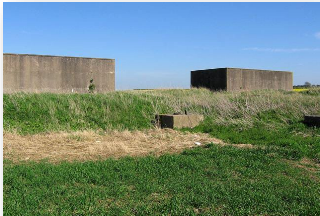
Figure 20: Thor Missile site, Former Melton Airfield
