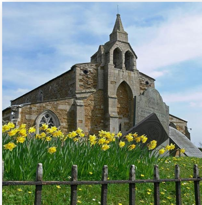
Figure 13: Grade I Listed Church of St James, Burton Lazars
